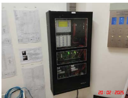
Fire alarm control panel
